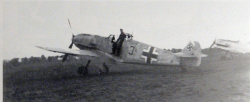
ABOVE: Two BF 109 Es of II (J)/Tr Gr 186 in early spring 1940. The aircraft in the distance has the standard early 1940 camouflage of black-green (RLM 70) and the rest of the aircraft carried a splinter pattern of dark-green (RLM 71) and RLM Grey (RLM 02) on the upper surfaces with light blue (RLM 65) on the fuselage sides and underneath. The aircraft in the foreground has a square canopy and is probably an E-3. The smaller than normal number 'Black 3' is outlined in white and the fuselage appears to have been given a light mottled overpaint of dark-green (RLM 71) and RLM grey (RLM 02).
