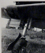
LEFT AND BELOW: Relatively few of these Caudron C.R. 71s were in service with the French Air Force and this one appears to have been captured intact. The interesting feature on this aircraft is that the wing guns have been housed in specially designed pod, just outside the inward retracting undercarriage. The pod allowed easy access to the guns and provided a larger ammunition storage facility.
